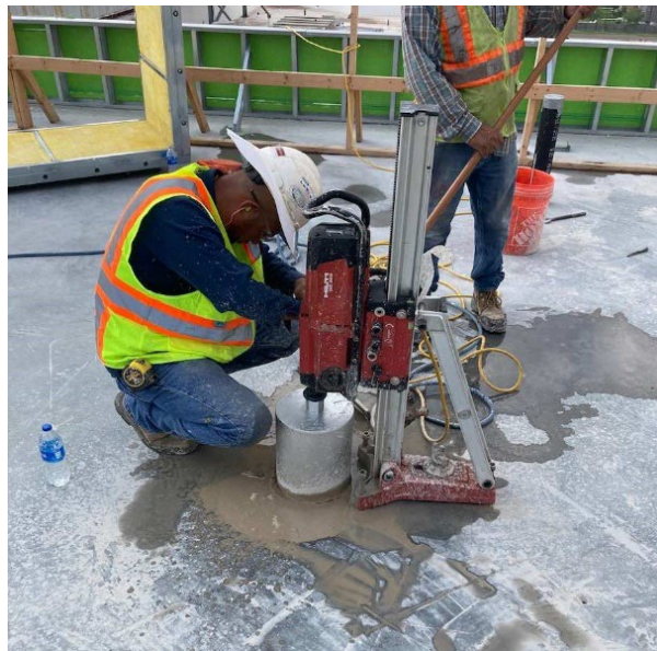
Figure 3 - Core Drilling
