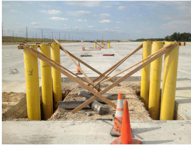
Figure 2 - Greenfield Bollard Installation
