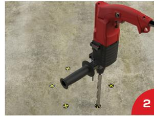
Remove base and drill six 16mm holes, 135mm deep. Clean out the concrete dust from the holes.
