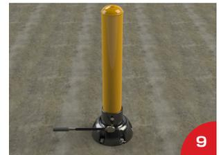
Tighten bolt so that it acts as a pin in the pipe hole. Firmly tighten all set screws to hold the bollard pipe in place. *Torque Spec: 50 ft-lb*
