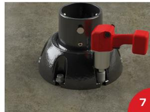
Tighten the concrete screw Anchors in a star pattern, compressing the elastomer and making the base flush to the concrete. Anchor heads must be tightened firmly, flush to base. *Torque Spec: 85 ft-lb*
