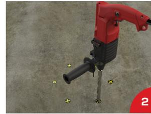
Remove base and drill six 3/4" holes, at a 5 1/2" minimum depth. Clean out the concrete dust from the holes.
