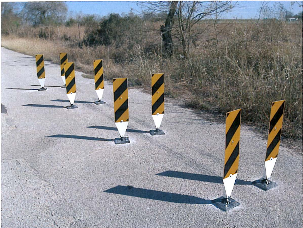
Photo #4 Object Markers installed, no impacts.
