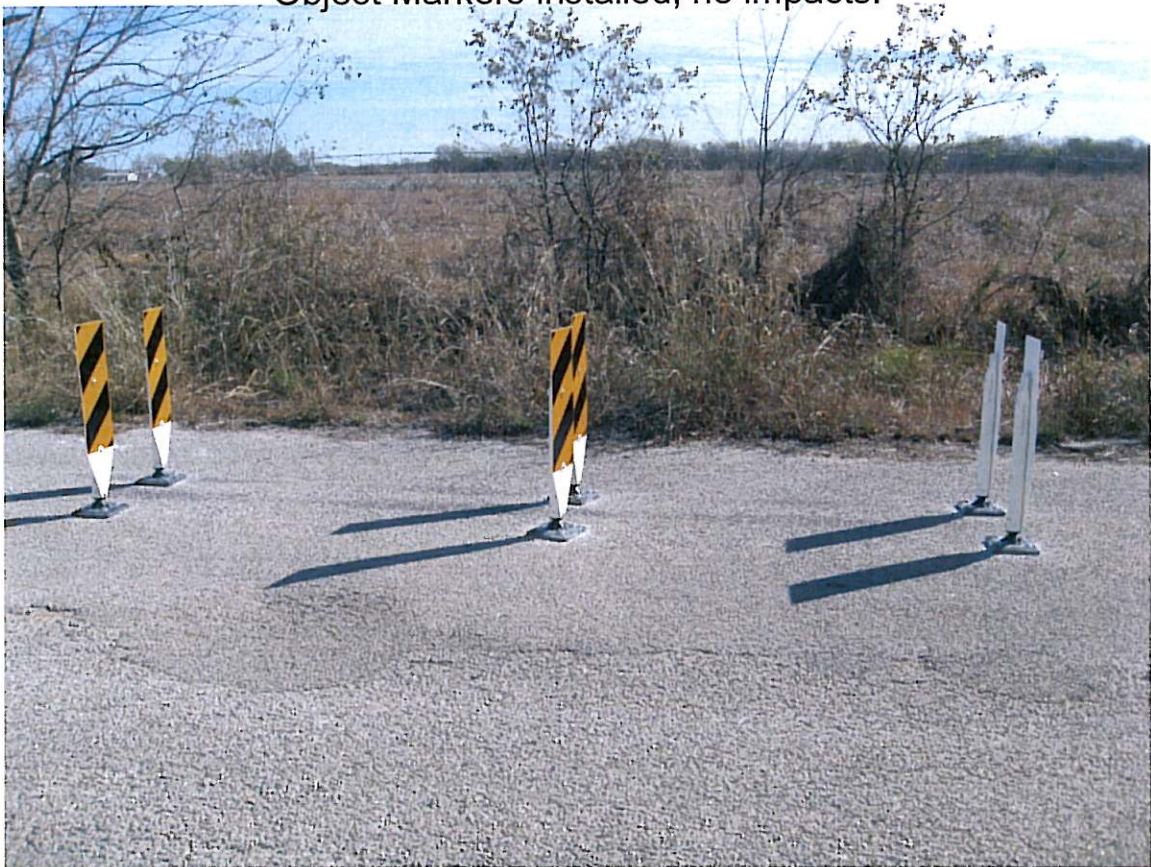
Photo #5 Object Markers installed, no impacts.
