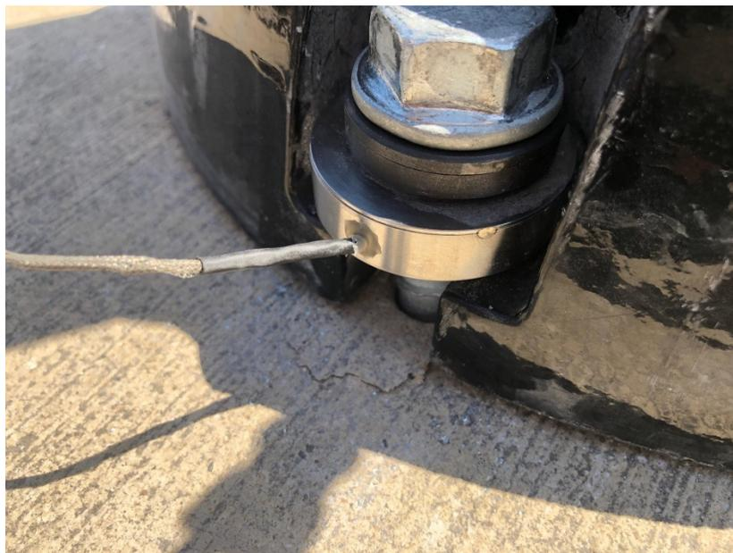
Figure 2 - Loss of Embedment at Load Cell
